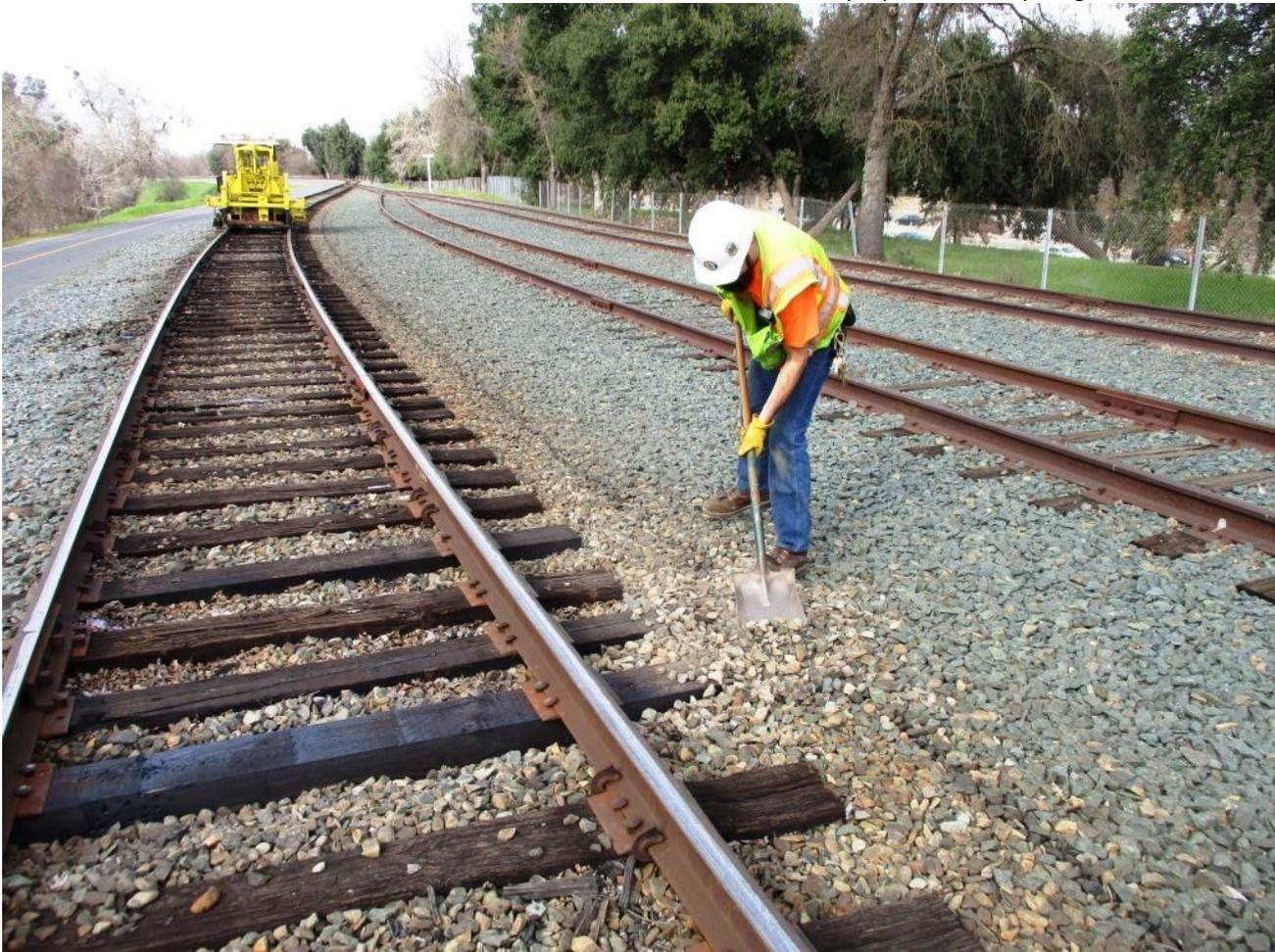
Matt works as a human ballast regulator to fill in holes that may be trip hazards
