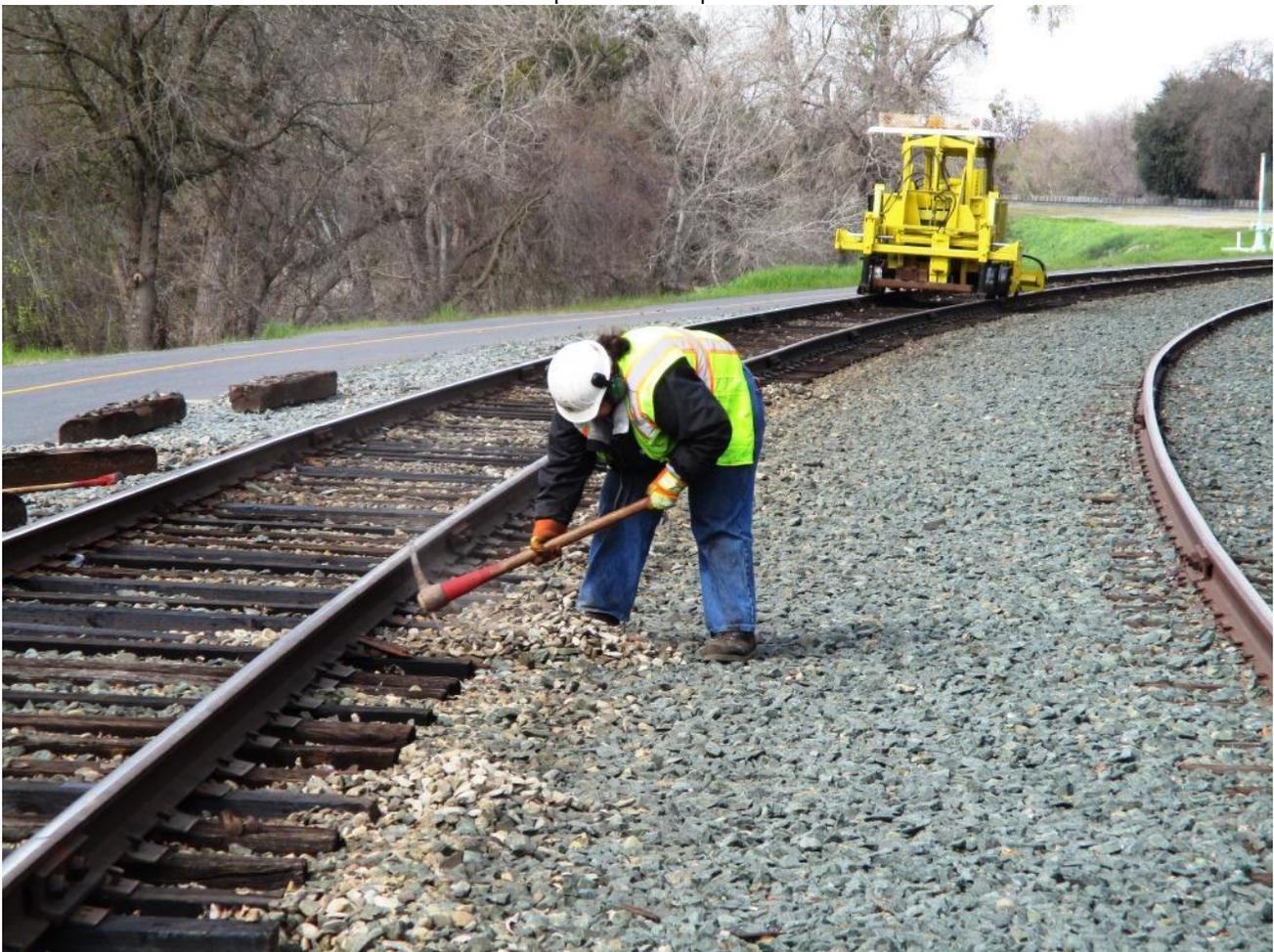
Heather spreads out the mounds of ballast rock which formed as a result of pushing the new ties under the rails
