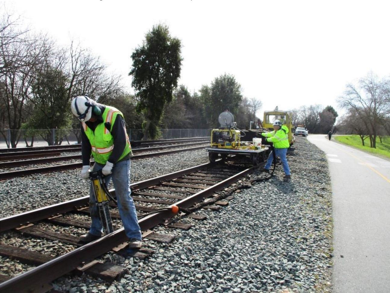
At Baths, Steve employs the hydraulic spike-puller to remove spikes on ties being replaced as Bill help by handling the hydraulic hose
